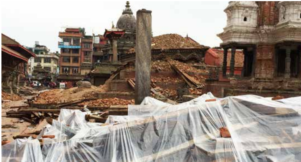
Top: Darbar square on second day, local stakeholders guarded day and night for security and safety. Photo: April 26, 2015. Bottom: All the wooden artifacts were covered with plastic sheets to protect from the rain. Photo: April 28, 2015.
