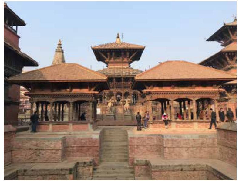
Top: Both Manimandapas collapsed in the earthquake. Photo: Suresh Lakhe. Apr. 27, 2015. Bottom: After rebuilding. Photos: Dec. 12, 2018.
