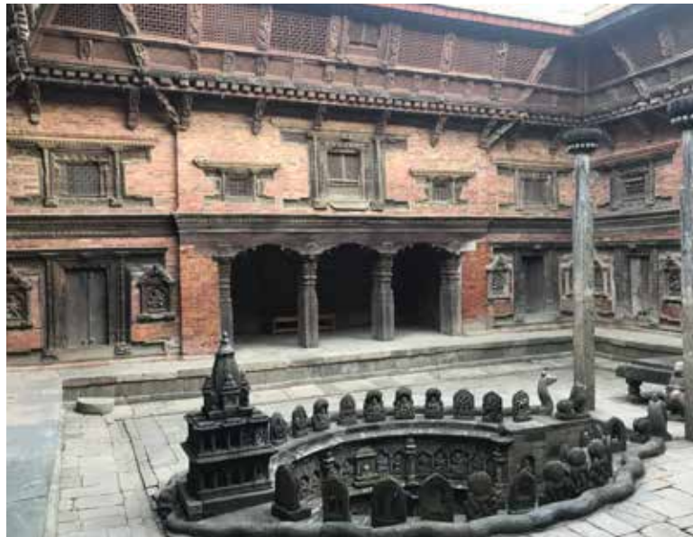
Top: Sundari Chowk East Wing after the earthquake. Photo: Apr. 27, 2015. Bottom: After rebuilding. Photos: Dec. 12, 2018.
